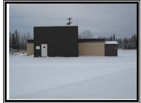
Building 633, the sewage treatment plant, which is slated for significant upgrades.
