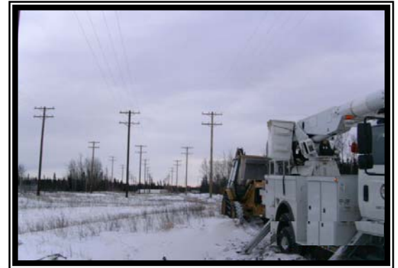
Construction of new electrical power lines at Fort Greely.
