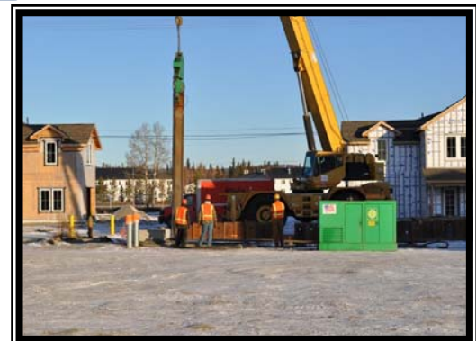
Alaska Groundworks installing sheet piling at Bear Paw Phase 1 at FWA.
