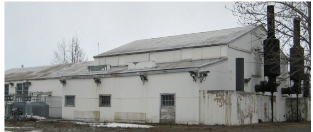
Pictured above is Building 772 scheduled for demolition.
